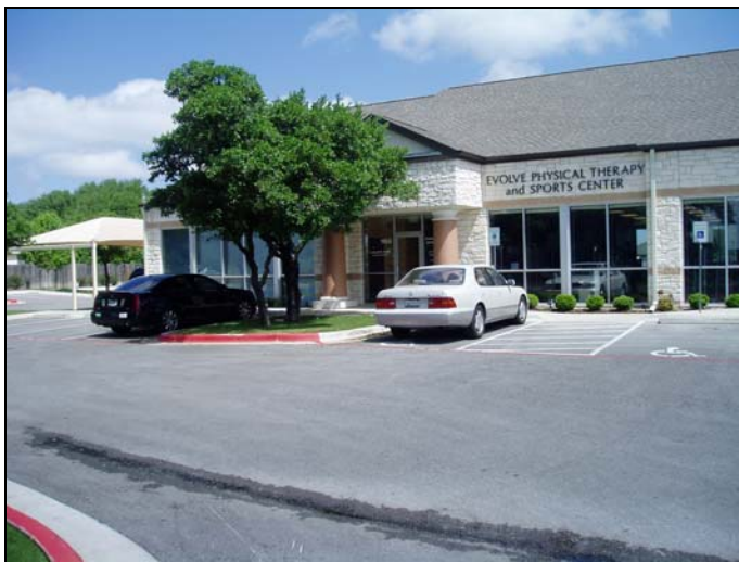
Front of Building
